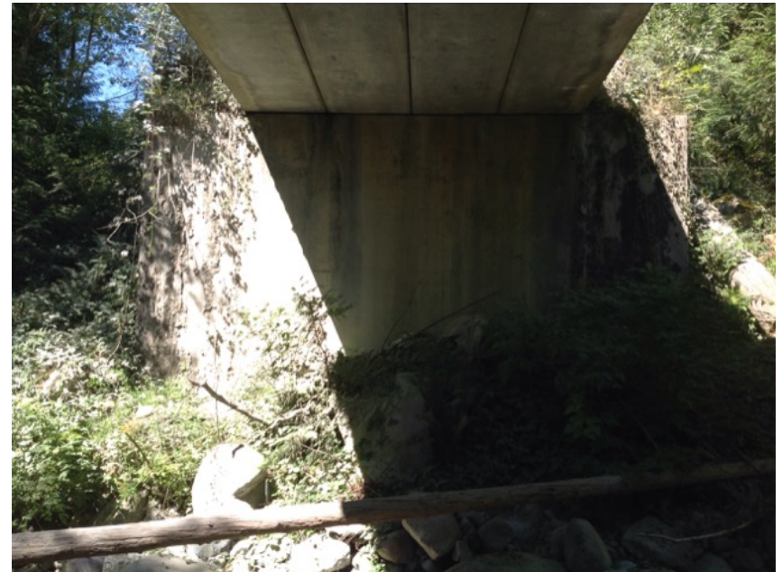
Right Bank Abutment when facing downstream
