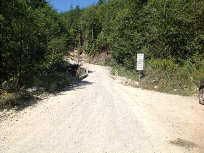
Approach from Left Bank when facing downstream
