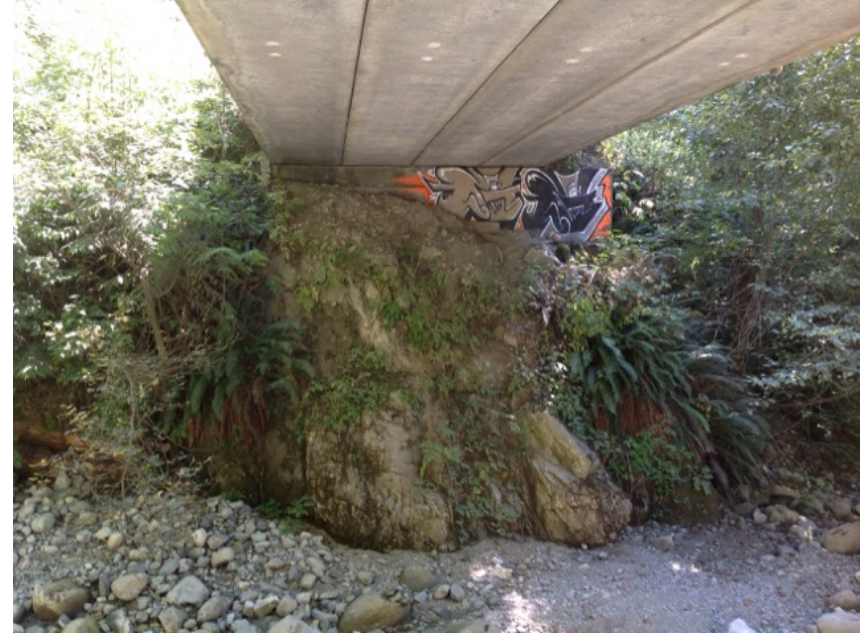
Left Bank Abutment when facing downstream
