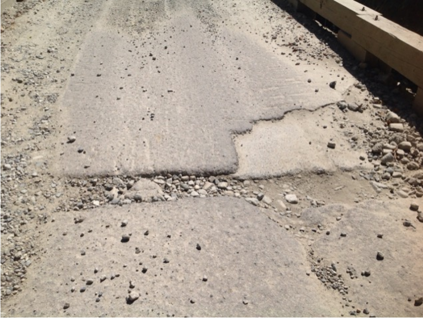
50mm asphalt overlay
